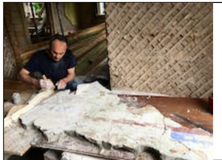
restoration work... 3.7 MiB
