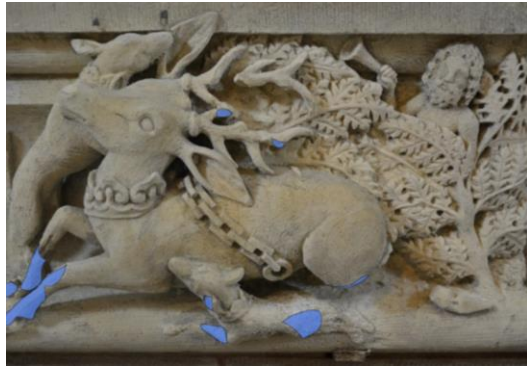
Recording areas of mortar consolidation
